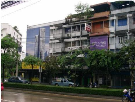
Figure 9: The same façade design with different alterations of the shophouses. The advertising billboard covers the whole façade units; some units are painted in different colors; windows are changed for different purposes.
