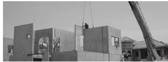
Fig 3 Precast concrete panels are used as loading-bearing structure for house construction.
