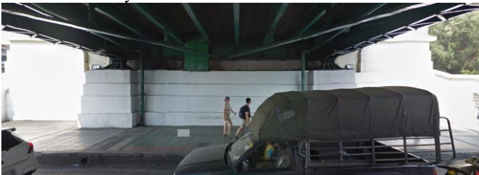
figure 22: site specific: memorial bridge NO.3
