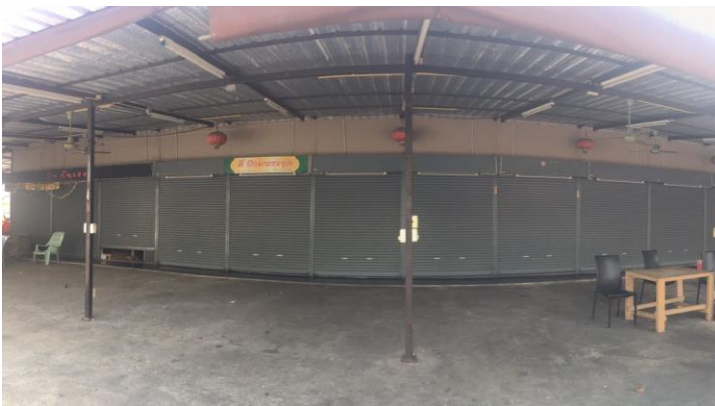
figure 25: tadindeang market new installation area
