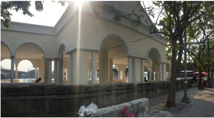
figure 20: site specific: memorial bridge NO.1
